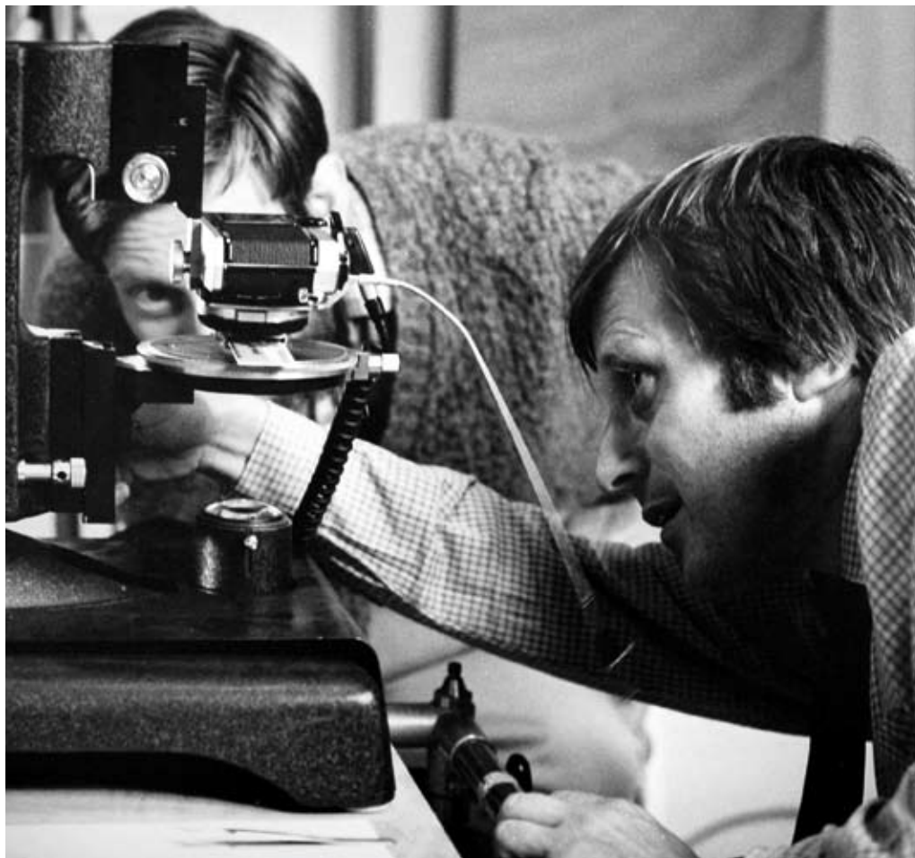
Fig. 15. TAKING MICROGRAPHS WITH THE LEEUWENHOEK MICROSCOPE AT UTRECHT During the original experiments with the Utrecht microscope the author was assisted by Dr Robert Frederick (left). The Leeuwenhoek microscope was lain on a specially-constructed holder made from plastic and mounted to the Olympus OM 2n 35 mm microscope. This was fitted on an early nineteenth century photomicrographic stand. The photographs figs 12 and 11 were with this device.
