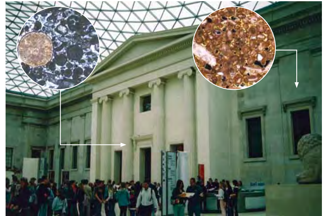
Fig. 5. The unexpected appearance of the new portico of a historic building, following construction with the wrong stone. The insets show the microscopical appearance of Anstrude limestone (upper left, field of view: 7 mm) and the Portland limestone (upper right, field of view: 5 mm).
