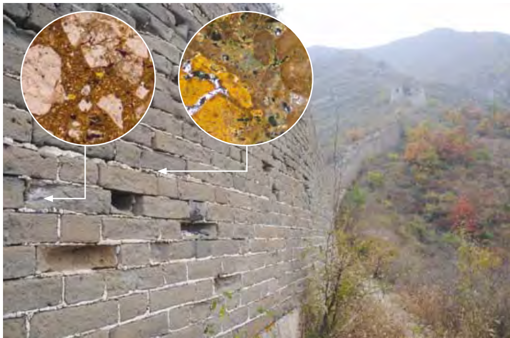
Fig. 8. The Great Wall of China at Panjiakou Reservoir, Hubei. The insets show the microscopical appearance of the brick (upper left, field of view: 1.8 mm) and lime mortar (upper right, field of view: 4.5 mm).
