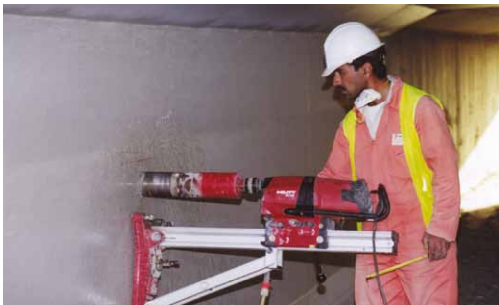
Fig. 1. Obtaining a concrete core sample from a concrete structure by diamond drilling.
