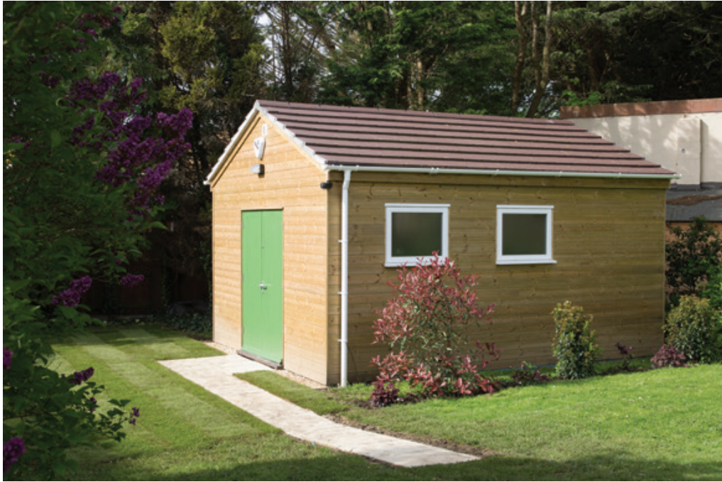
Figure 2. Exterior view of the laboratory
